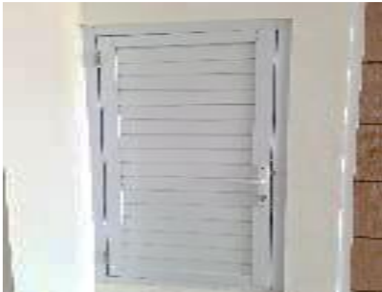
Gambar 8. Finishing pintu shaft
