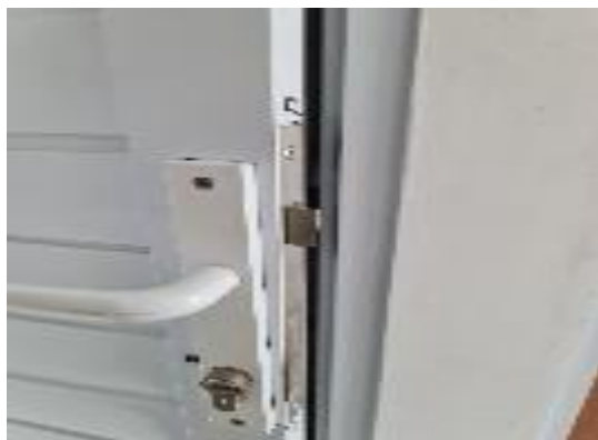
Gambar 8. Finishing handle pintu shaft
