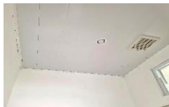
Gambar 7. Finishing plafon kamar
